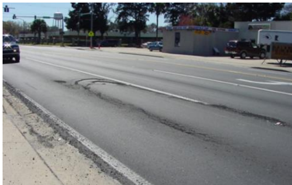
(a) slippage failure
