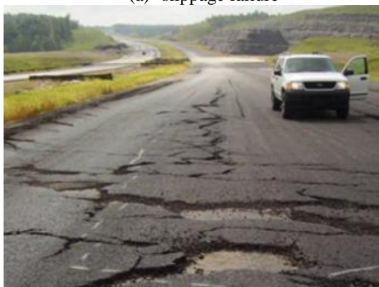
(b) Delamination
