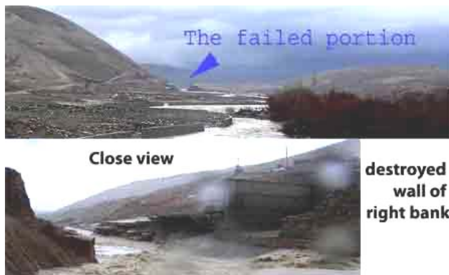
Fig.12: Broken dam's wing at the right bank of Chaq Chaq valley
