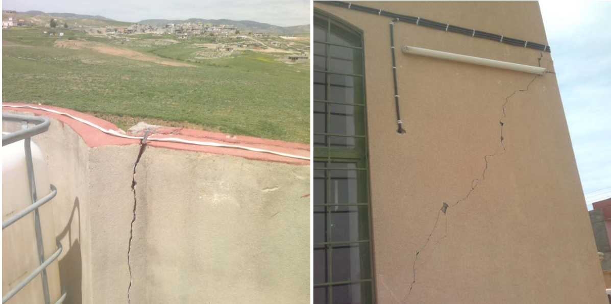
Fig.8: Crack in a fence of a house (left) and a wall in recently built mosque (right), in Shaikhan town
