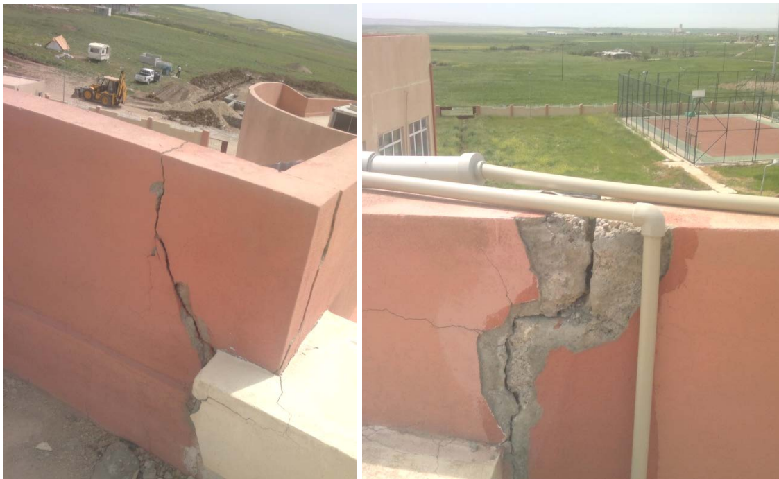
Fig.9: Cracks in a roof fence of the youth center in Shaikhan town
