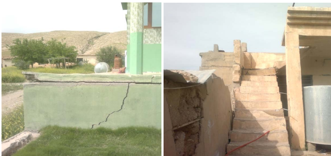
Fig.6: Two houses in Beristiq village showing cracks in concrete foundation ( left ) and wall ( right )
