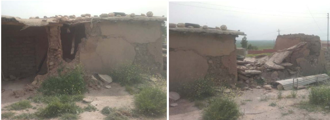
Fig.5: Collapsed mud huts in Beristiq village
