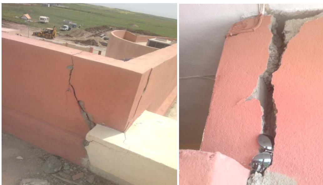
Fig.7: Cracks in roof fences of a house in the Youth Centre in Shaikhan town
