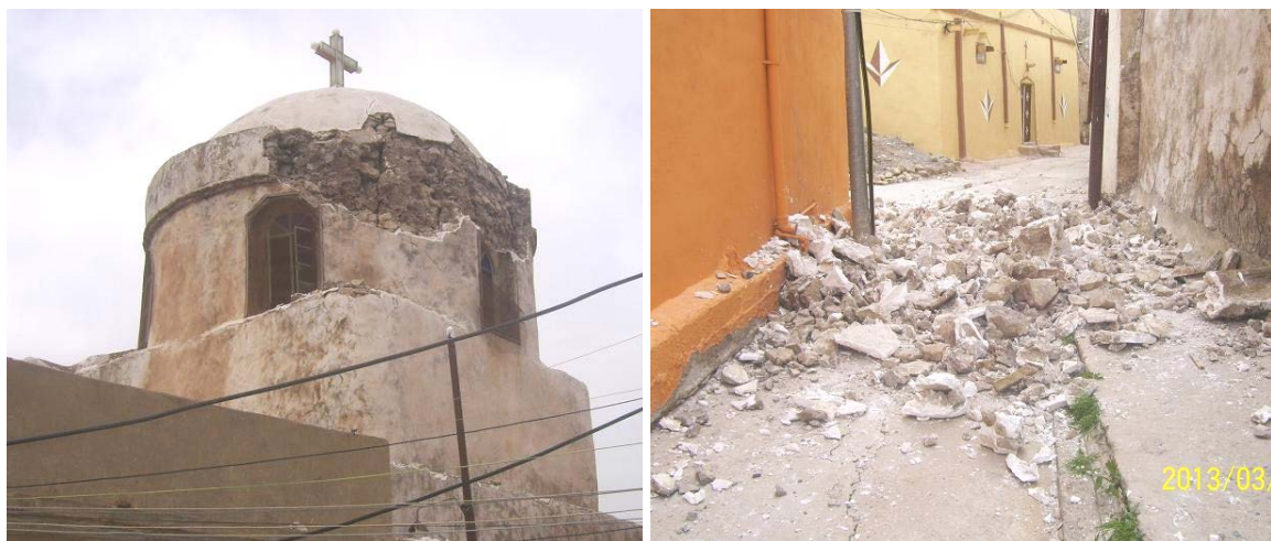
Fig.3: The cracked dome of Mar Yacoub Church (left), the fallen plaster pieces (right) in Tell Asqaf village
