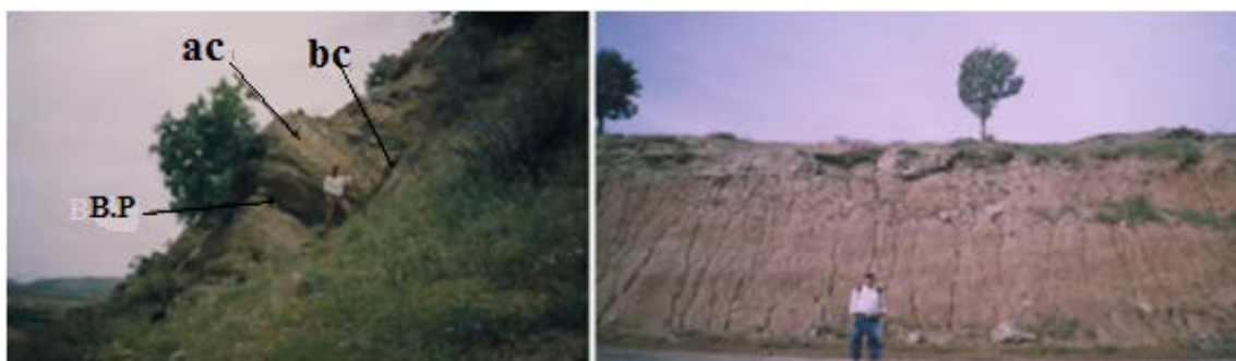
Fig.4: Side and frontal views of sites 18 and 20 respectively, of potential plane sliding
