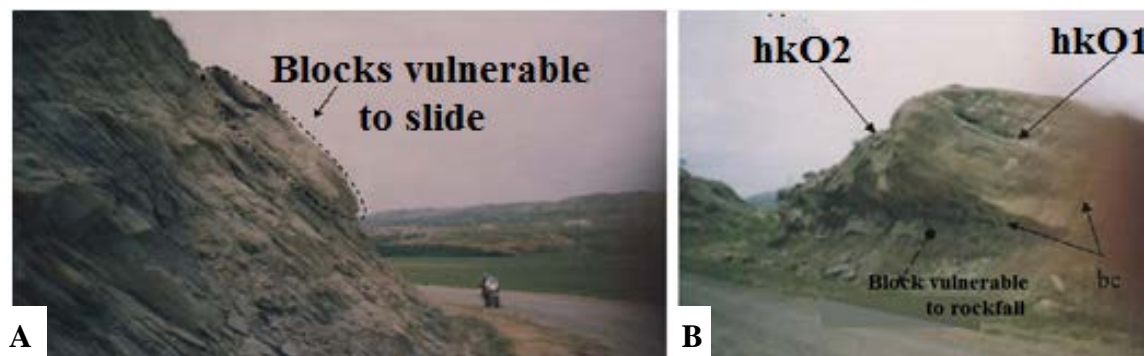
Fig.3: Side views of sites 11 (A) and 14 (B); showing the blocks vulnerable to rockfall on Mirawa road
