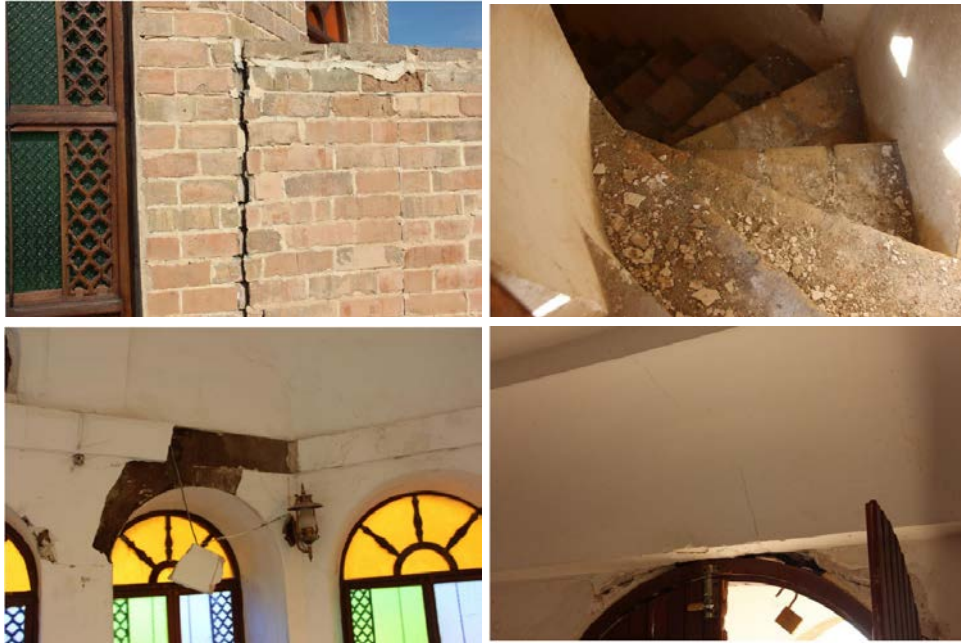
Fig.9: Cracks in a roof, a wall, and the fallen plaster pieces in the second floor in Sherwana castle
