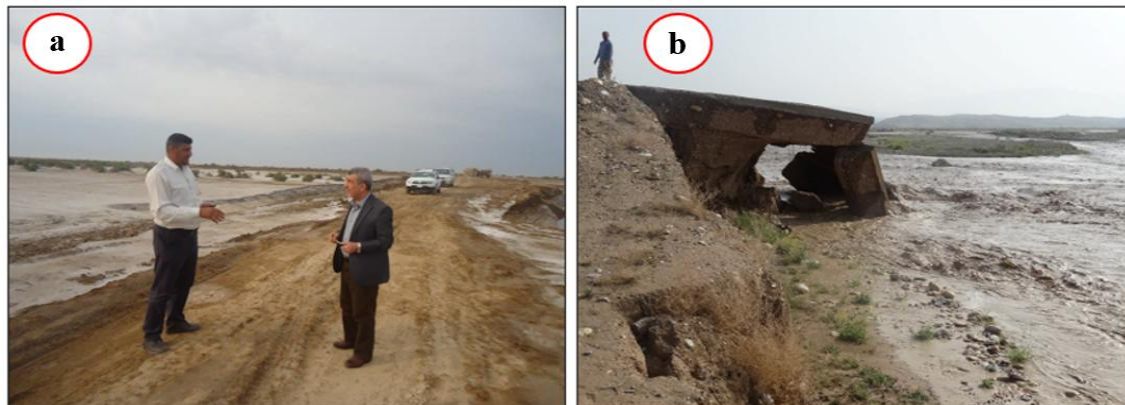
Figure 10. Flooded streams in the eastern part of Iraq (Mesopotamian Plain). a) An eroded embankment, b) A damaged culvert.
