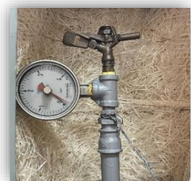
Fig. 5 The iron stand for the sprinkler inside the cylindrical tank.
