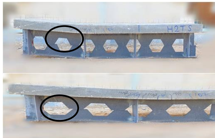
b) Failure of H2TS
