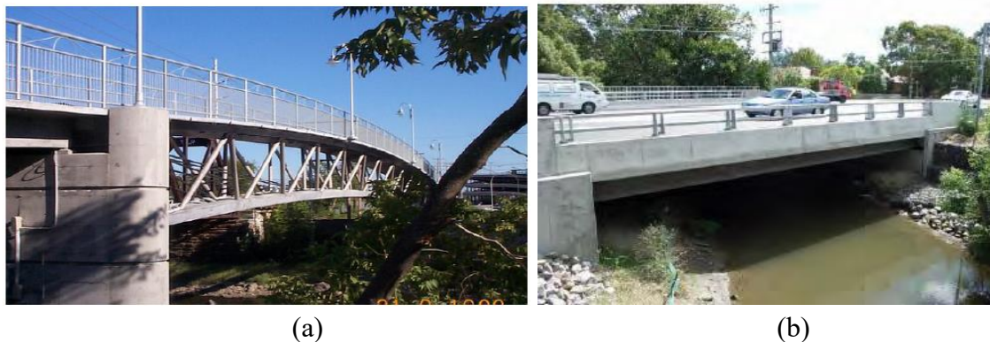
Fig. 2. a: Sherbrooke footbridge and b: Shepherds Creek bridge
