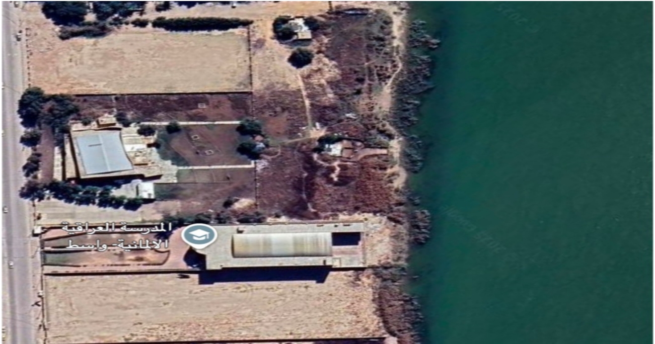
Figure 2. The section of the Tigris River that Al-kut Barrage.
