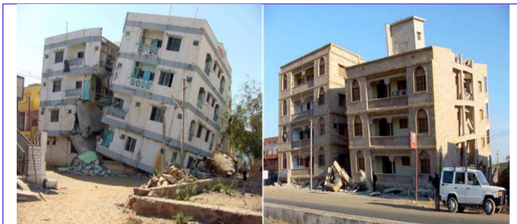
Fig. 5. Seismic Buildings with Open Ground Storeys - RC frame structures with open ground storeys collapsed after 2001 (Bhuj in India) Earthquake [27].
