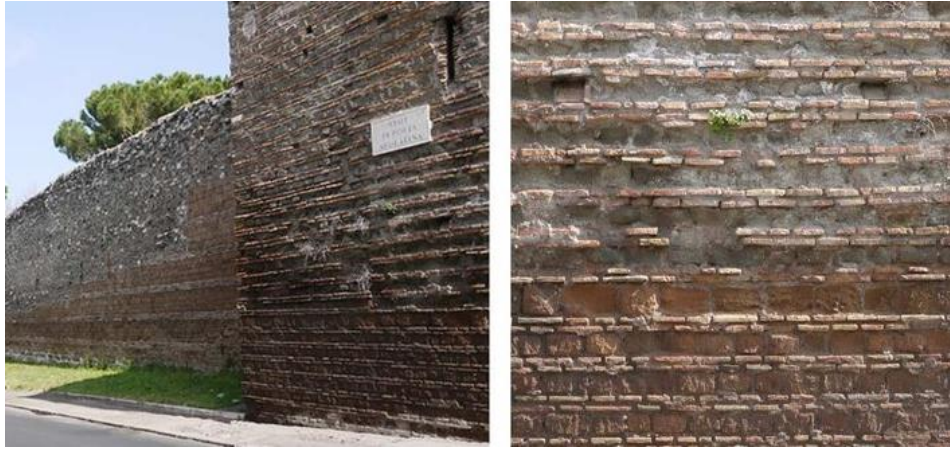
Fig. 6. Brick and stone construction on the Aurelian walls, Rome, 3rd century AD [21].
