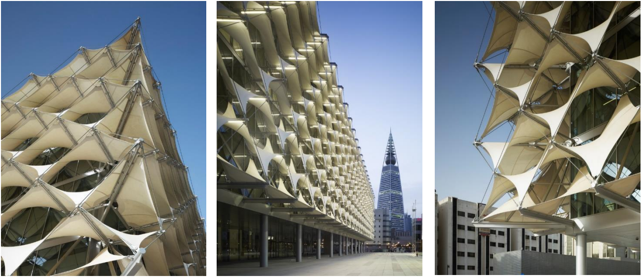
Fig. 10. Details of the diamond-shaped textile canopies, which were taken from the idea of the Arab tent, but in a unique and advanced form that is in harmony with current progress [28].
