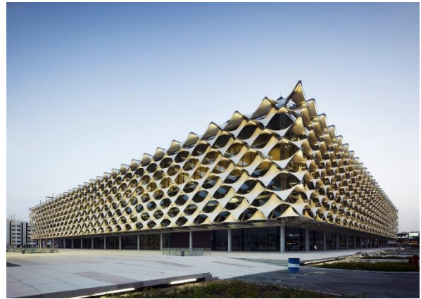
Fig. 11. The exterior facade of the new building, which is controlled by the opening and closing of the textile elements [29].
