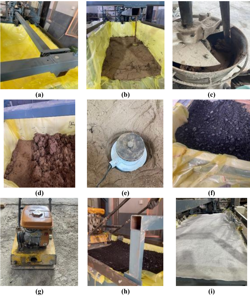
Figure 5: (a-i) Scaled model of the flexible pavement construction
