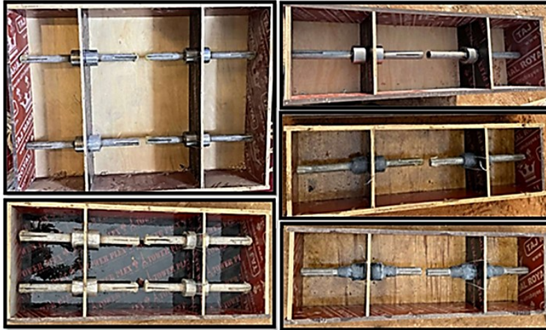
Fig. 3. Preparing the molds before pouring
