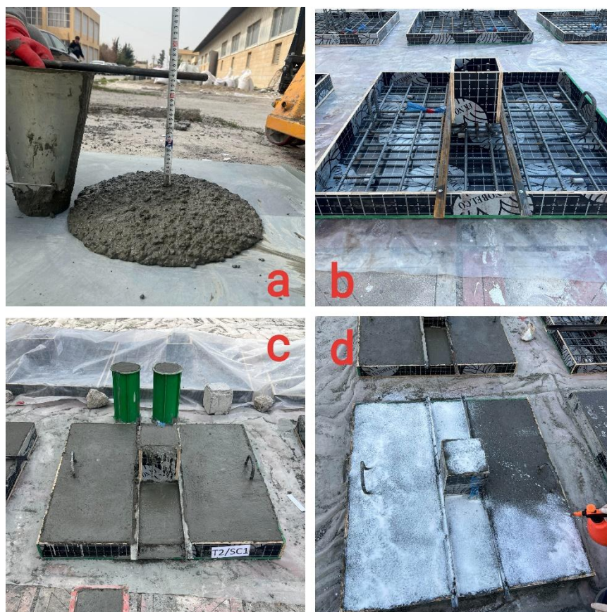
Figure 2: Slab's casting configuration (a) slump of mix, (b) preparing mold, (c) casted sample, and (d) spring curing material
