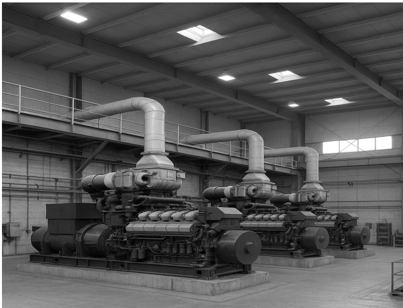
Figure 1: MAN 18V32/40 engines installed for power generation in an Iraqi industrial facility, representative of the equipment analyzed in this study[3].
