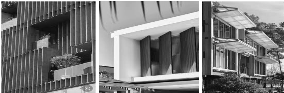
Figure (6): Different shapes of horizontal and vertical solar refractors on building facades.
