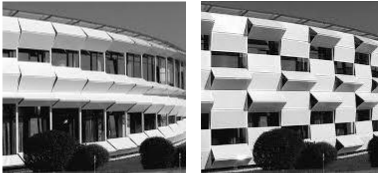
Figure (7): Kiefer building facades
